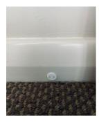
For timber treatment testing, we remove face plates from some of the power or light sockets mounted on external walls. Through the inside of the enclosures, we drill into a stud and extract timber drillings which we test for timber treatment. The face plates are replaced and there is no external evidence that we have taken samples.
