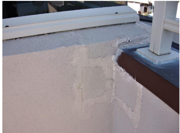
Invasive Testing Cut-Out – Exterior
